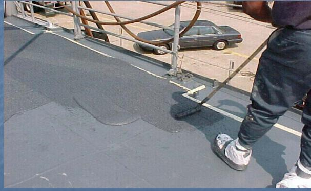
POUR A "RIBBON" OF NON-SKID ON THE SURFACE 2' TO 3' LONG AND APPROXIMATELY 1' TO 2' WIDE. ROLL MATERIAL IN ONE DIRECTION ONLY, IN SLOW STRAIGHT STROKES PULLING MATERIAL TOWARD YOU WITH A MODERATE AMOUNT OF PRESSURE ON THE ROLLER HANDLE. DO NOT OVER-ROLL TOO MANY TIMES OR PRESS DOWN TOO HEAVILY.
