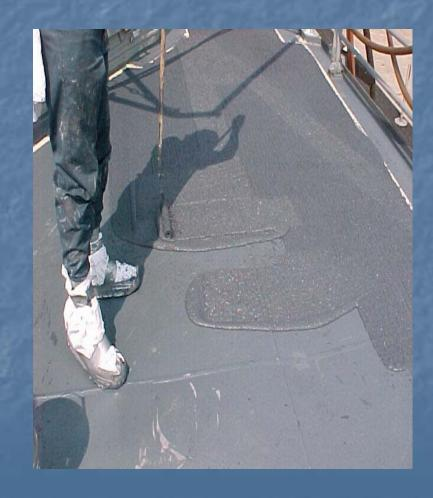
PULL AND DISCARD MASKING TAPE WHEN THE NON-SKID IS CURED ENOUGH FOR FOOT TRAFFIC.
